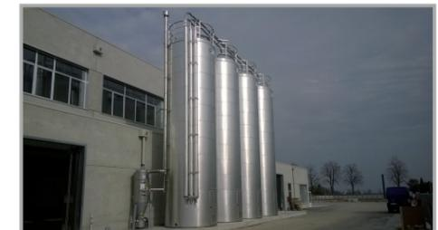
SILOS DI STOCCAGGIO COIBENTATI CON IMPIANTO DI FILTRAGGIO CENTRALIZZATO
