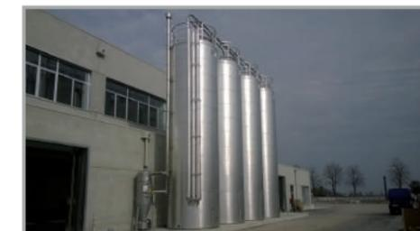
SILOS DI STOCCAGGIO COIBENTATI CON IMPIANTO DI FILTRAGGIO CENTRALIZZATO
