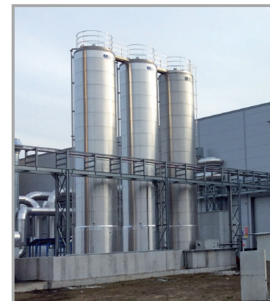
SERBATOI SU GONNA DA 90 MC RISCALDATI E COIBENTATI PER OLII PLASTIFICANTI 90 M 3 HEATED AND INSULATED SKIRTED TANKS FOR PLASTICISER OILS
