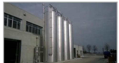
SILOS DI STOCCAGGIO COIBENTATI CON IMPIANTO
